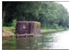
Bunker in Bree
