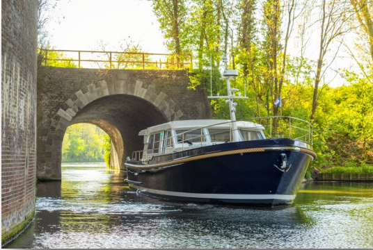
Tunnel am Bassinhaven
